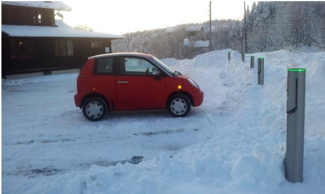
Figure 6: 10 new charging points installed at Frognerseteren, in the hills outside Oslo.
